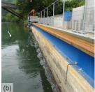
Fig. 3: (a) Vortex tube connecting the headrace channel with the residual flow reach (Photo: VAW) (b) Horizontal bar rack for fish protection (Photo: VAW)
