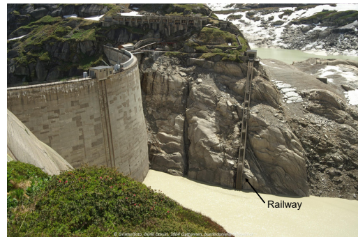
Fig 3: Lowered Grimsensee in 2006 with Spitalamm dam on the left and existing railway. (Photo: KWO)
