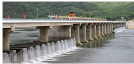
Figure 1: Van Phong Dam, Vietnam
