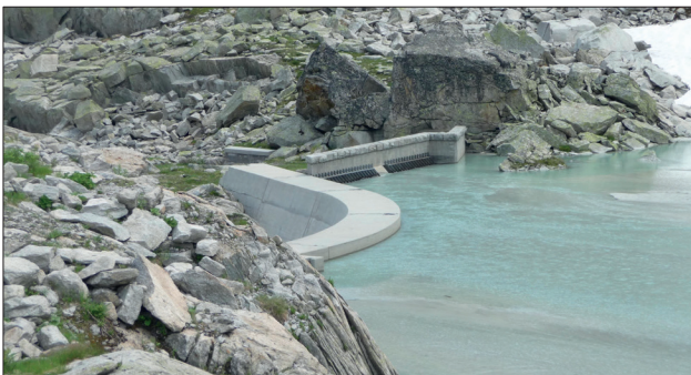
Figure 2. The Bächlibach dam which diverts the water into the Bächli gallery. The water intake is equipped with a trashrack to avoid big stones to enter the gallery. The capacity of the water intake is 7.5 m 3 /s.
