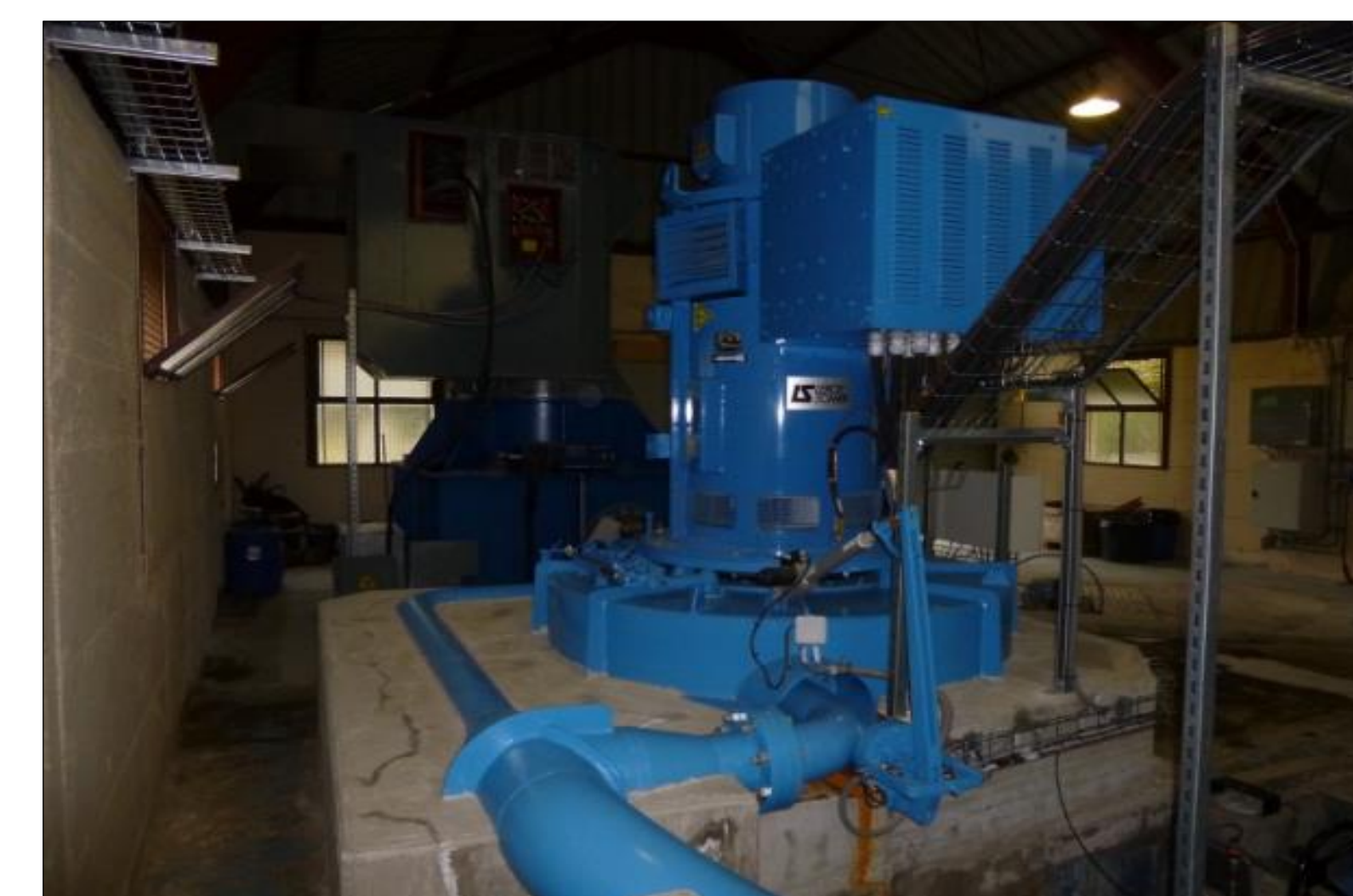
Figure 4. Picture of a Pelton turbine with two injectors from the power plant Le Lauzet in France (Cerec Engineering):
