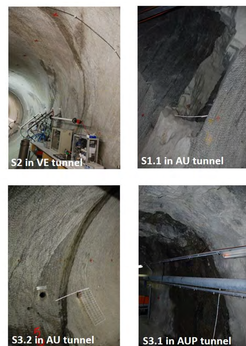
Figure 1. ISC experiment from south-west isometric view with three main intersecting sub-vertical fracture zones. Some intersection of these shear zones with the existing tunnels are shown on the right hand side.
