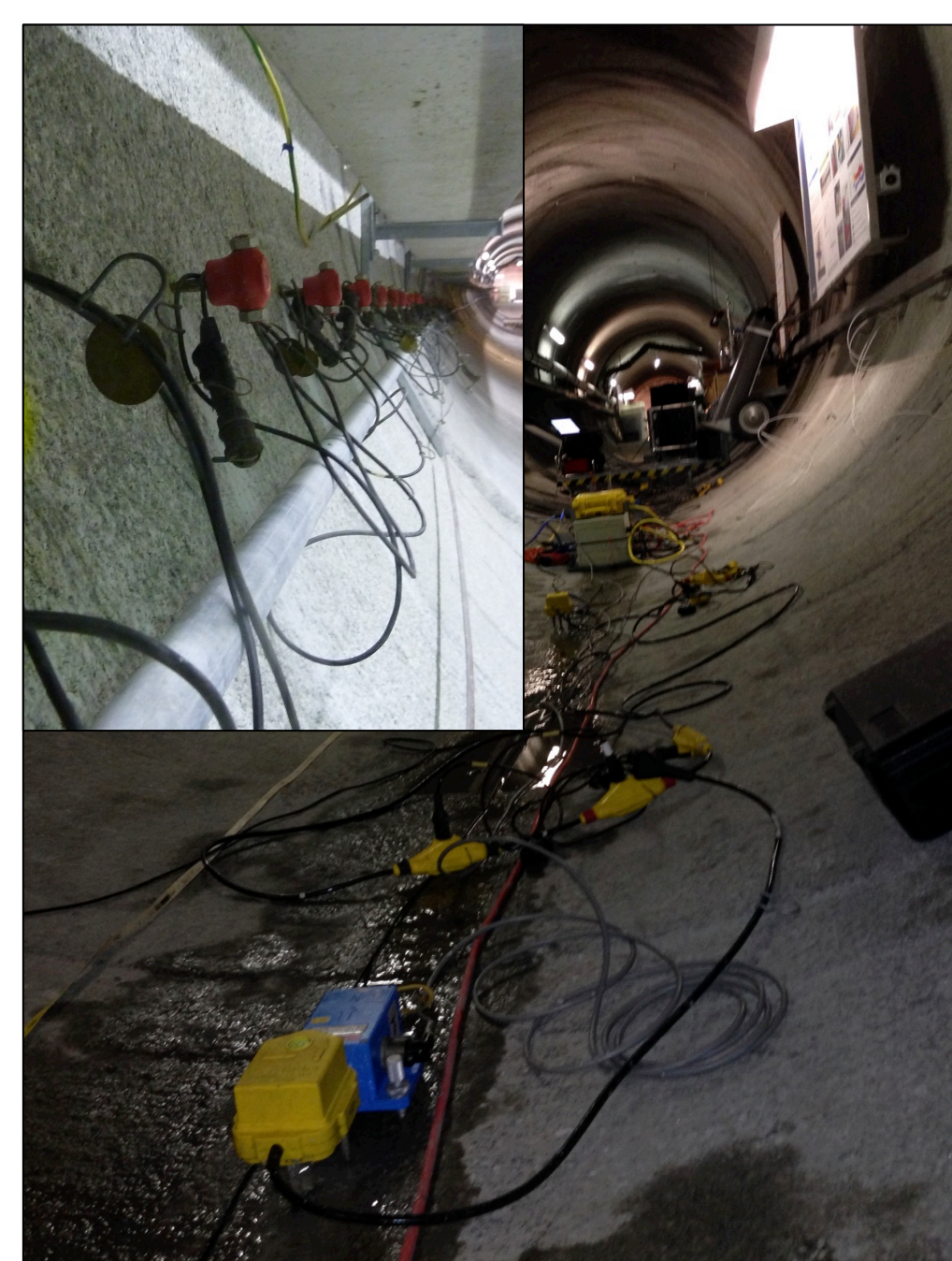
Geophones on the tunnel floor and the tunnel walls
