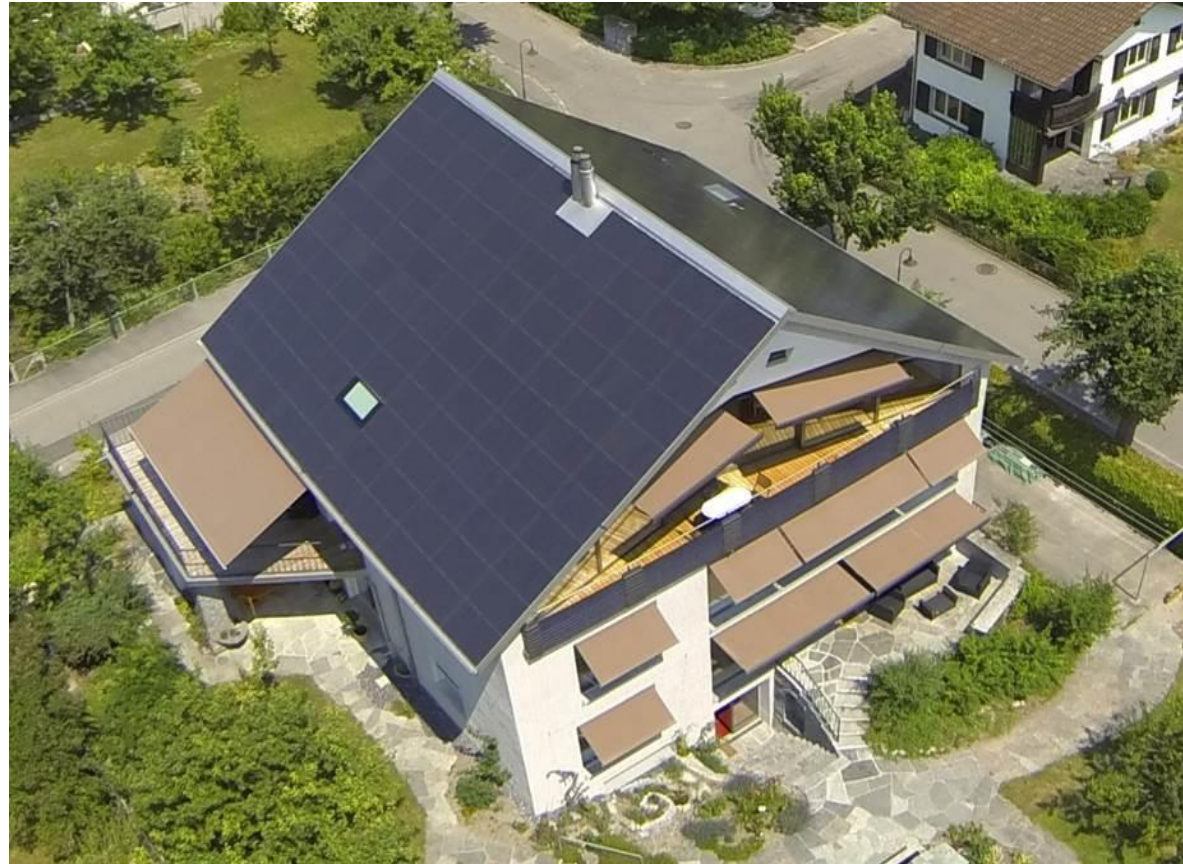
Roof integrated PV installation in East-West configuration
