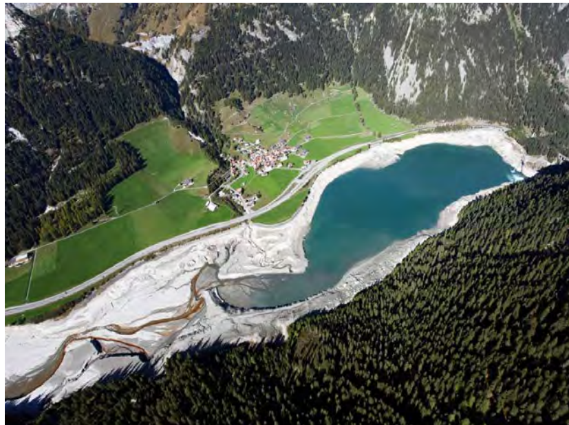
Sedimentation of Sufers reservoir, Switzerland (photo courtesy of Kraftwerke Hinterrhein AG)
