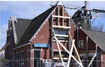
A condemned and shored-up cafe. Photo: Graham Dockery
