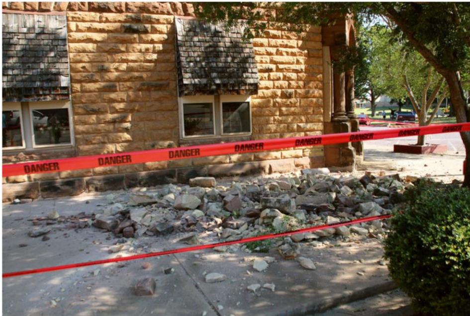
Stonework fell to the sidewalk at the corner of Sixth and Harrison Streets in Pawnee, Okla., after a 5.6-magnitude earthquake struck the area on Saturday morning. Lenzky Krehbiel-Burton/Reuters
