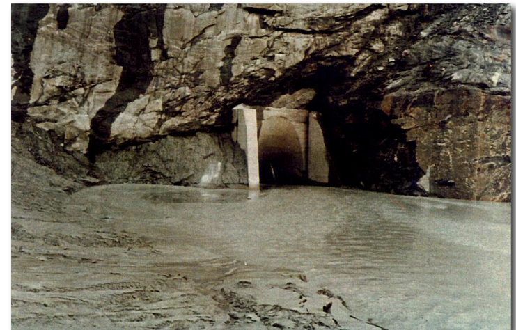
Sediments in front of the bottom outlet during emptying in May 1985
