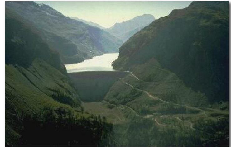
Mauvoisin arch dam in Canton Wallis
