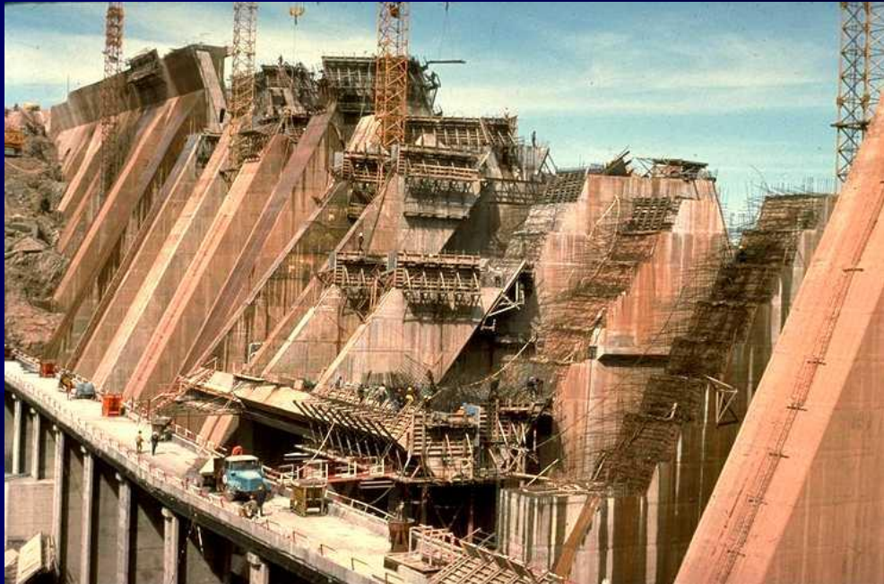
Al Massira Dam under construction
