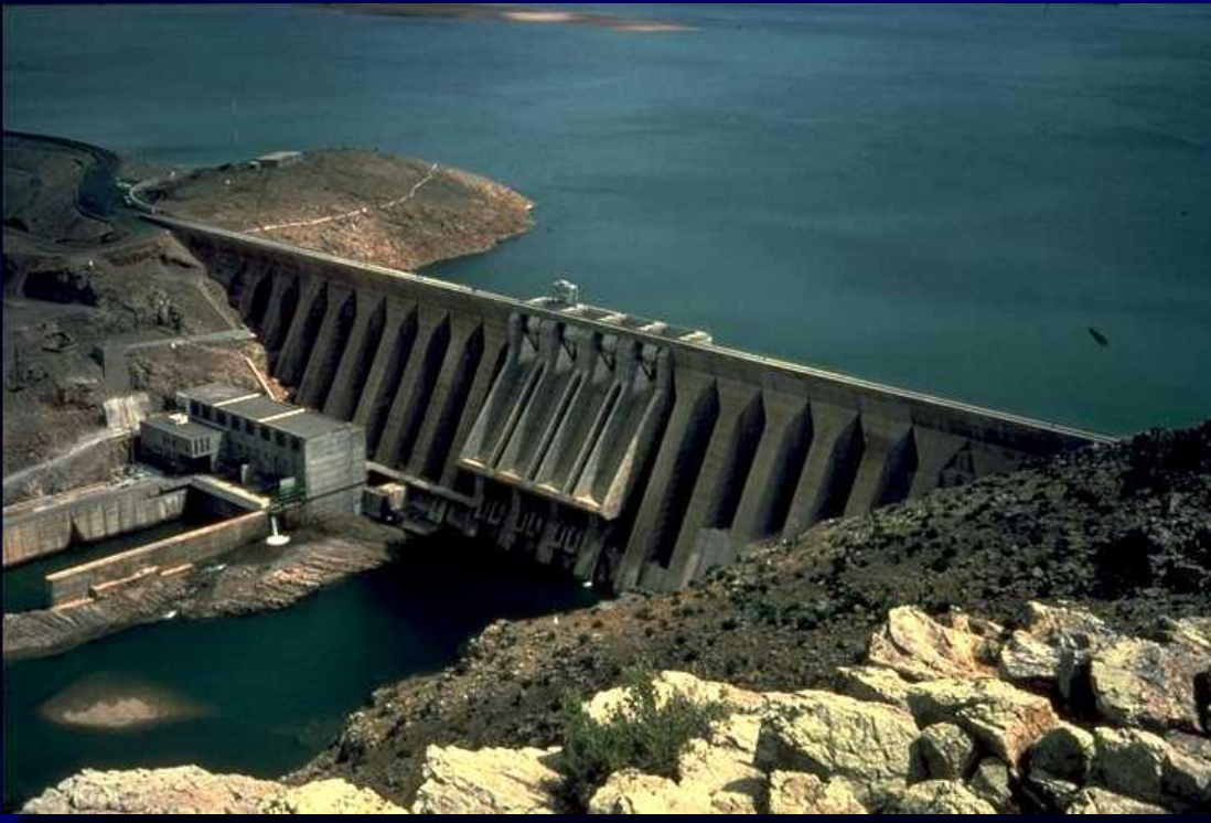
Concrete buttress dam, Al Massira, Morocco
