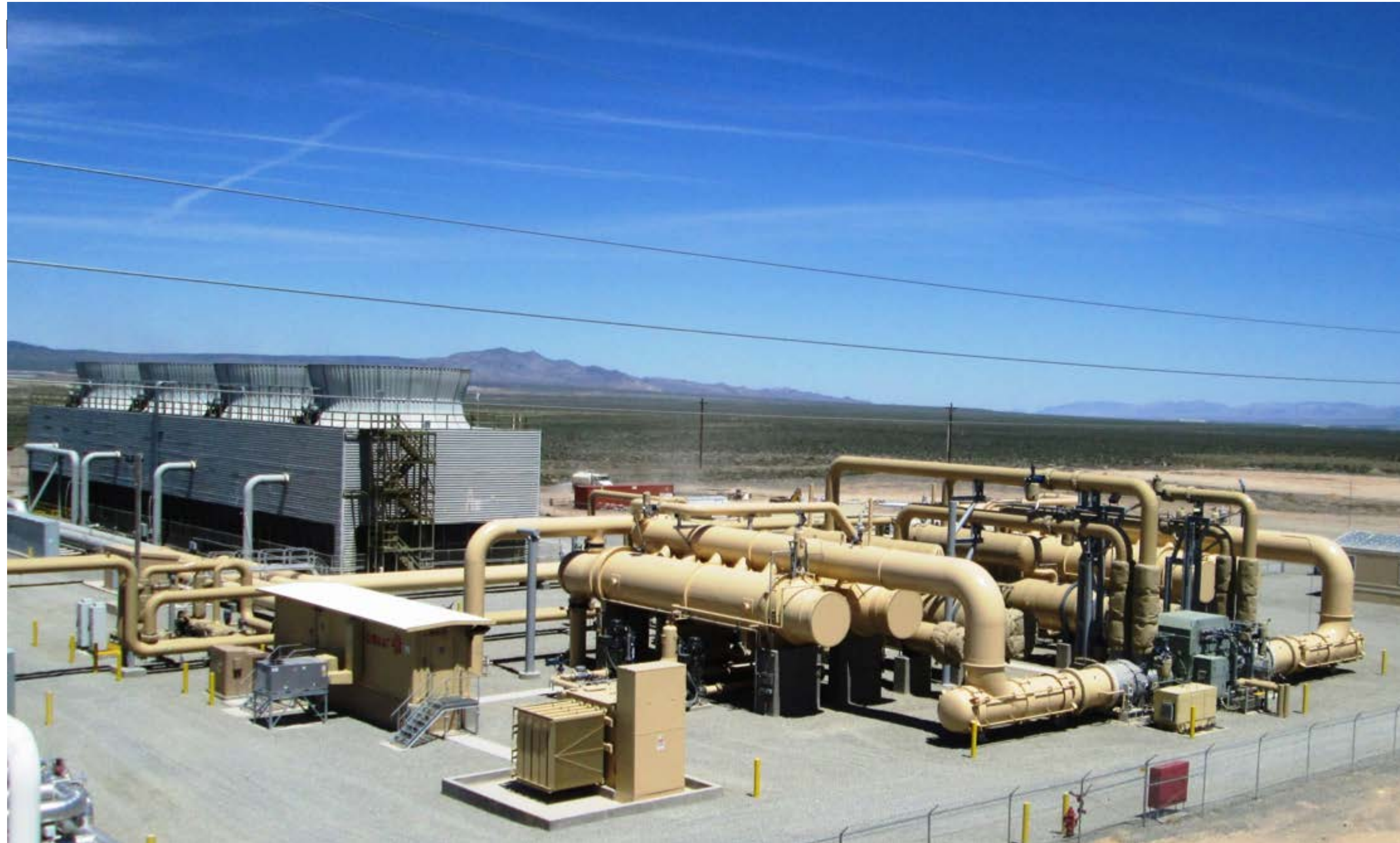
Thermo No. 1 at Milford: 10 MW Binary geothermal power plan
