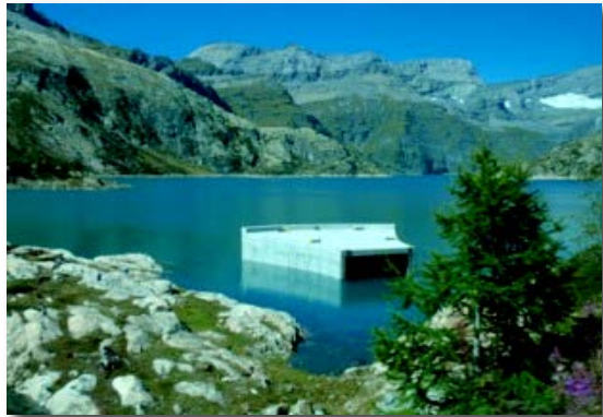
Pumped storage scheme Nant de Drance: New intake at Emosson reservoir (Schleiss July 2011)
