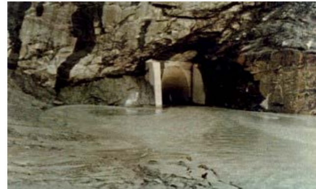
Sediments in front of the Mauvoisin bottom outlet during emptying in May 1985
