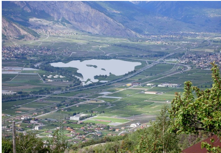
SYNERGIE Multipurpose project on Rhône River
