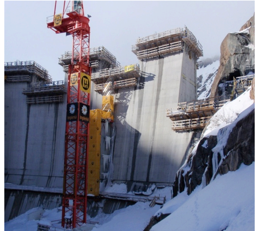
Nant de Drance pumped storage scheme: underground powerhouse excavation and Vieux Emosson dam heightening (Schleiss November 2013)
