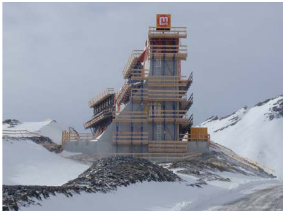
Muttsee Gravity Dam under construction
