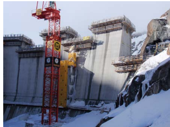
Vieux Emosson Arch Dam under construction
