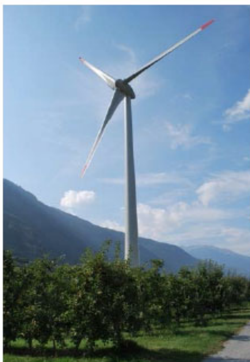
2 MW wind turbine, 5 GWh/a RhôneEole Martigny, 2008
